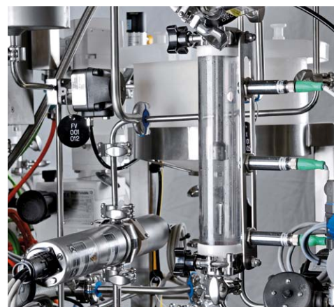
Bubble trap with level switches
